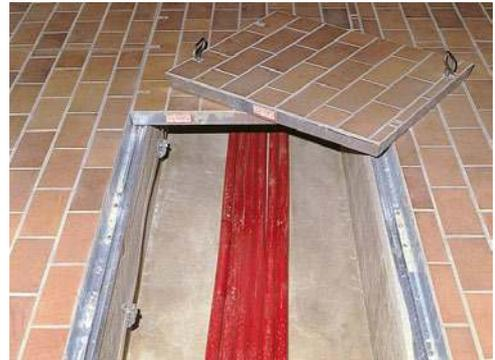
**Detail: Multi-part cover for cable duct**
